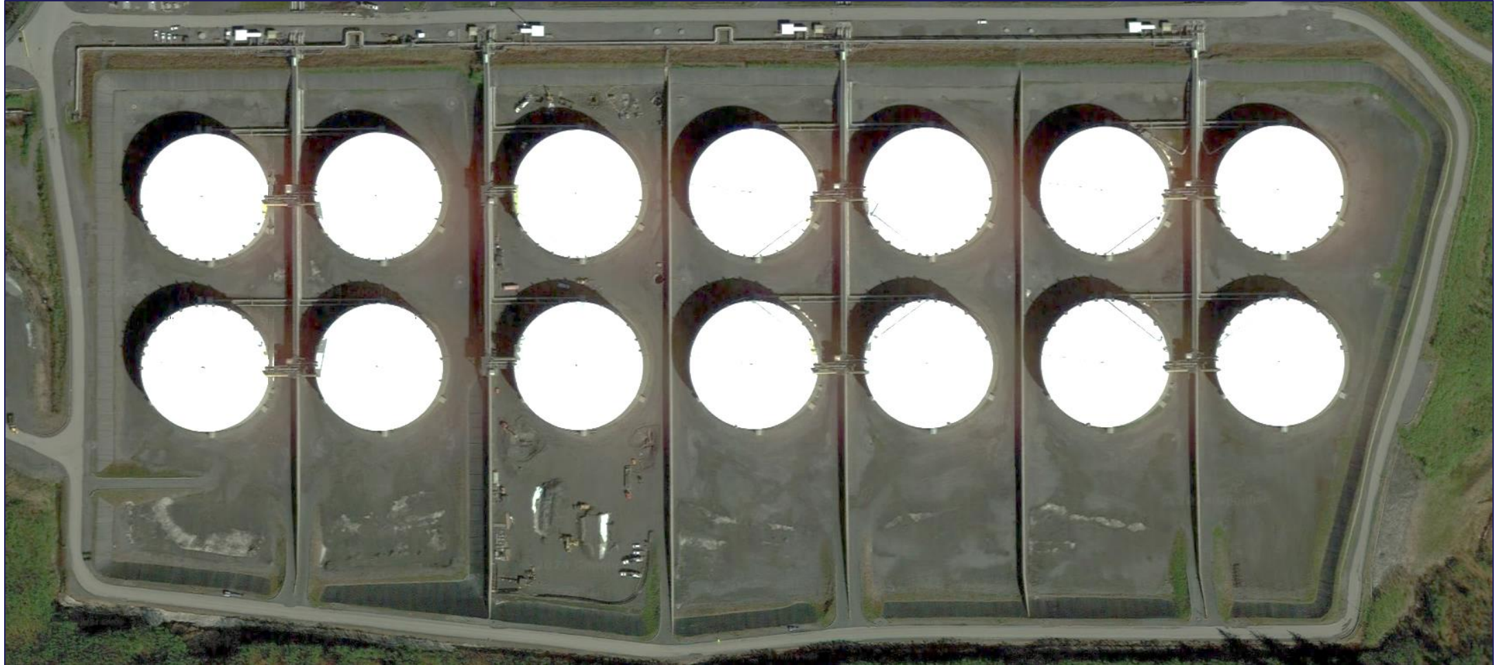
VMT East Tank Farm
