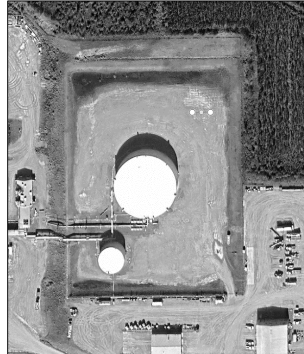
TAPS Pump Station 5
