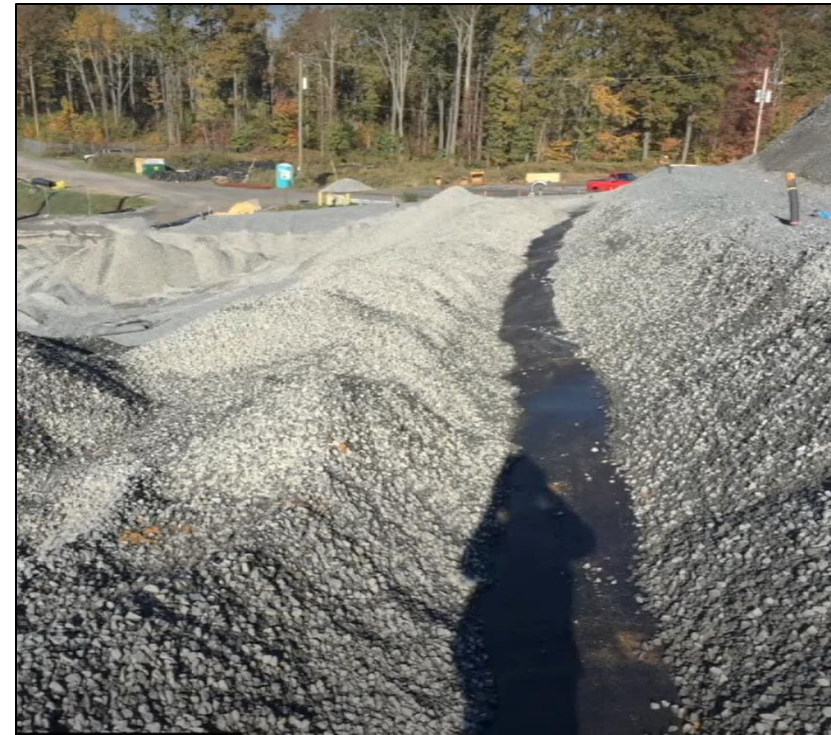
Example of ELL isolation trench (not at VMT)
